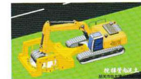
挖掉管内泥土 Digging the soil inside the pipe
